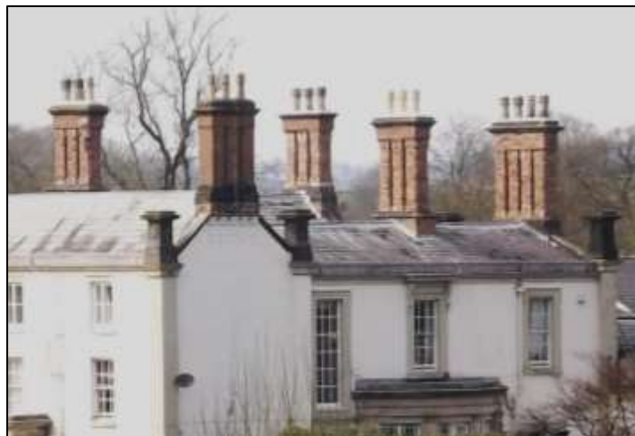
Figure 16: Dog-toothed eaves, castellated chimney pot and array of moulded brick chimneys at Hilderstone Hall
