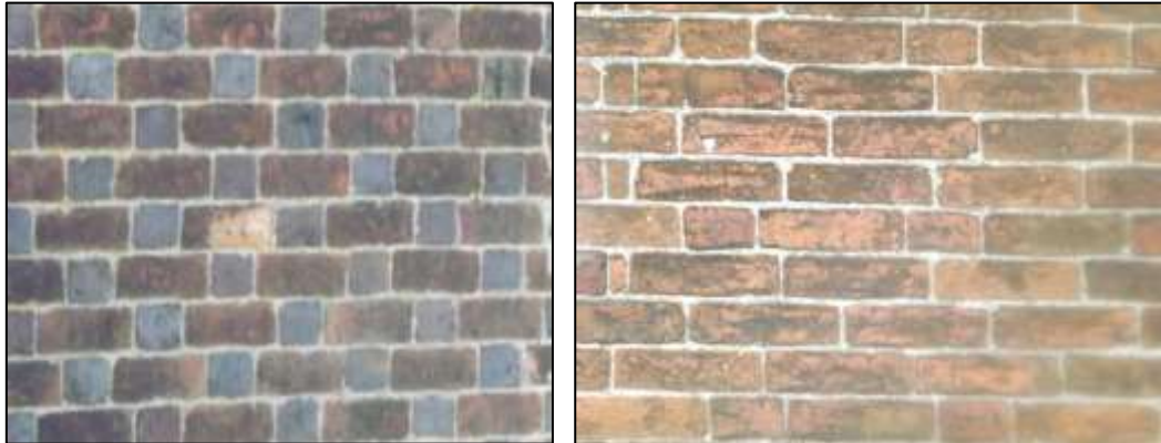
Figure 9: Alternating red and blue bricks in a Flemish bond creates a chequerboard effect at Vernon Cottage. Most buildings use bricks made of local orange clay in a simple Flemish garden wall bond.
