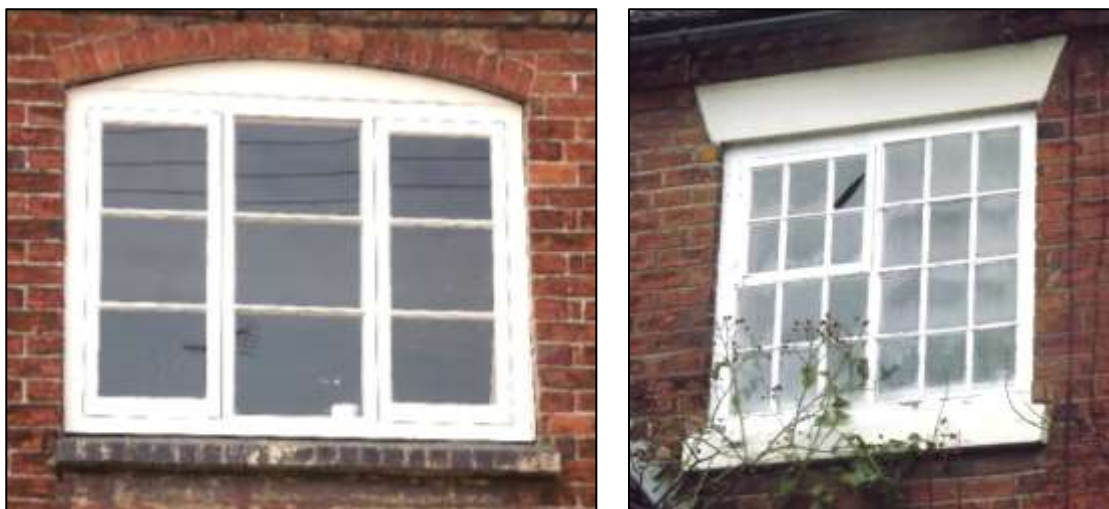
Figure 13: Variants of painted timber side opening casement windows.
