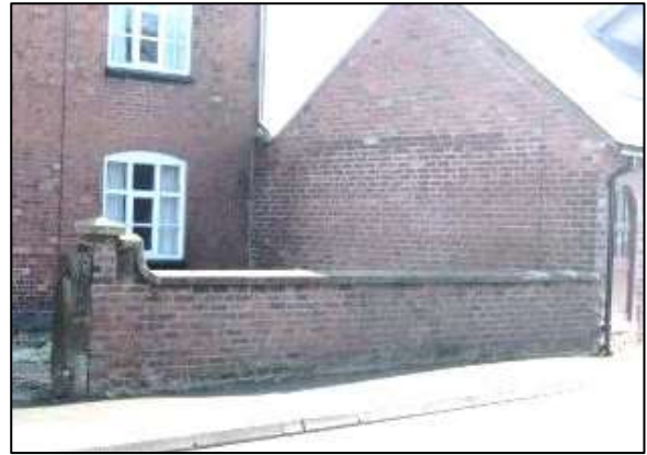
Figure 17: Variety of brick boundary walls with a variety of brick or stone copings
