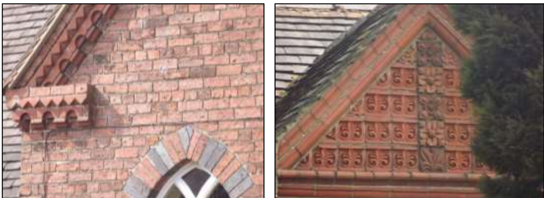
Figure 10: The use of moulded terracotta bricks and tiles, and polychromatic brickwork, at The Gables and the former Methodist Chapel.
