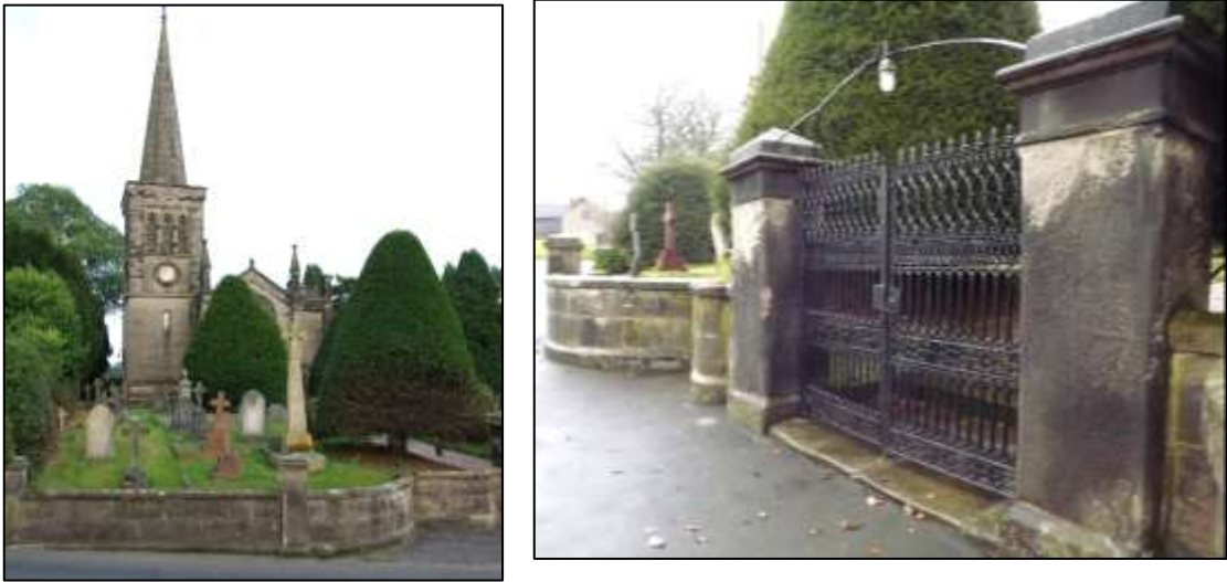
Figure 24: Christ Church and its independently listed wrought iron gates and gate piers
