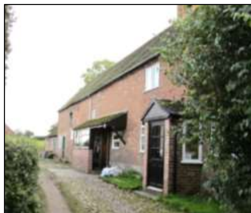
Figure 47: Converted agricultural buildings at Hill Farmhouse and Brook Farm, and Yew Tree Farm, a former agricultural building of Yew Tree Farm
