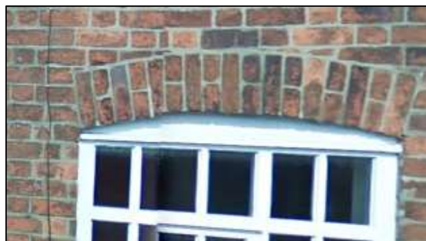
Figure 11: semi-circular brick arch over fanlight at Lower Farm house, and variations of the segmental arched window head.
