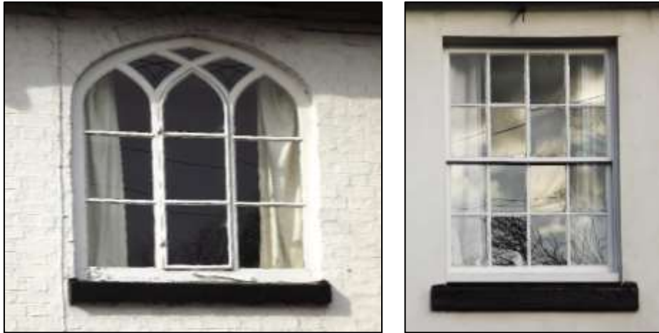
Figure 14: Gothic pointed arch casement at the School House, and typical Georgian sliding sash window within deep reveals.
