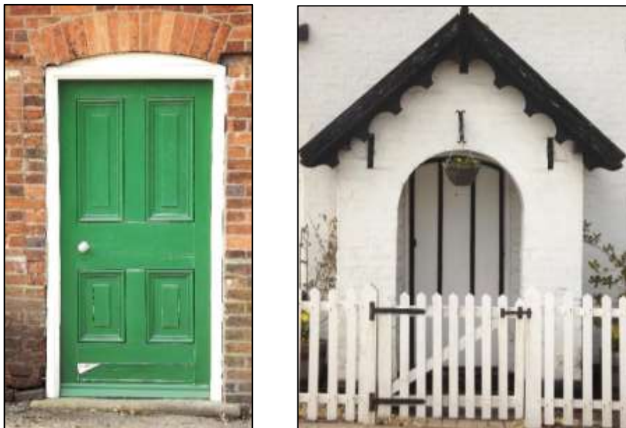
Figure 15: Victorian four-panelled door with well-defined moulding, and battened door within porch at The School House
