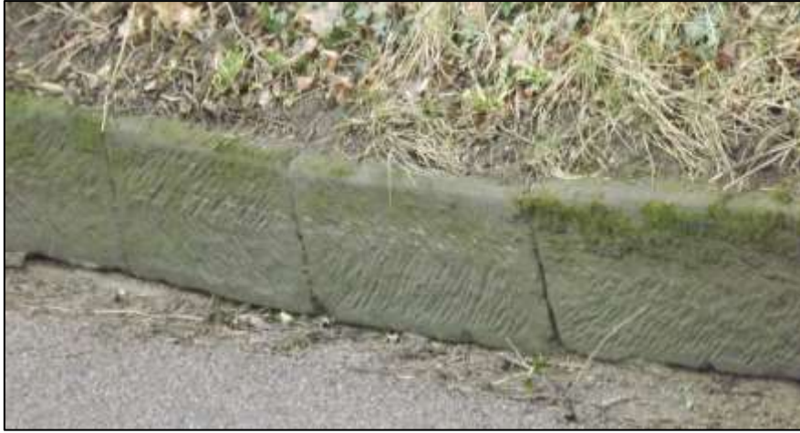
Figure 19: Tooled ashlar stonework bounding Cresswell Road
