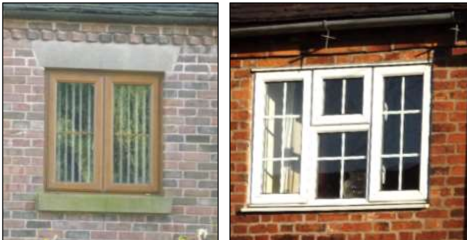
Figure 76: Examples of storm-proof casements, use of upvc and top opening casements. Positioning the windows forward in line within the brickwork accentuates the non-traditional form of glazing.
