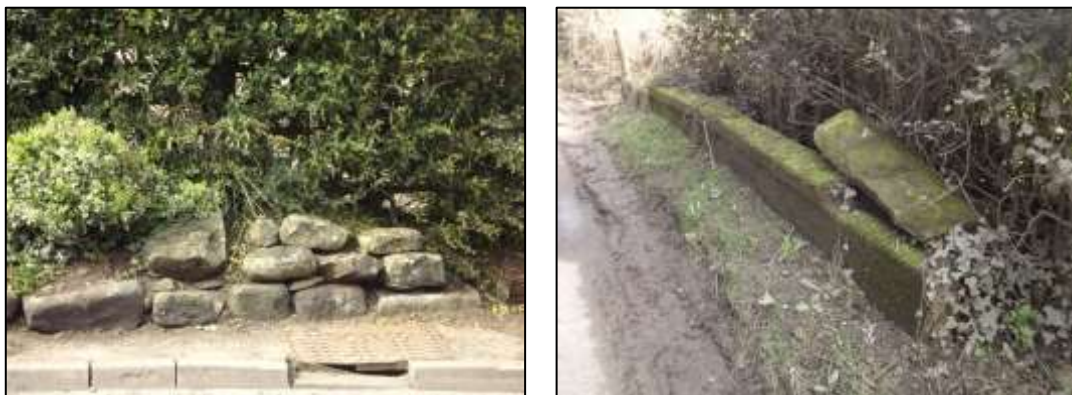
Figure 72: Condition of stone boundary walls
