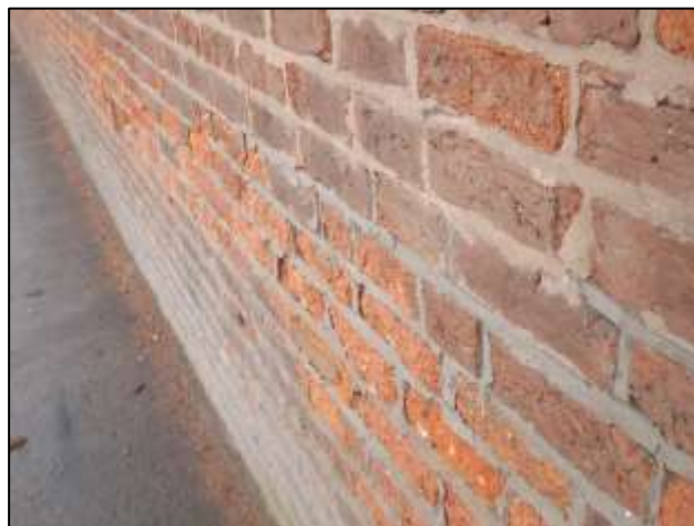
Figure 74: Example of a hard cement-based mortar causing erosion of soft historic brickwork.
