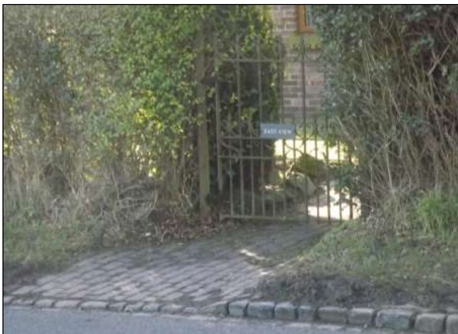
Figure 50: Where the stone sets of the highway kerb meet with historic brick pavers this adds character and detail to the street scene.
