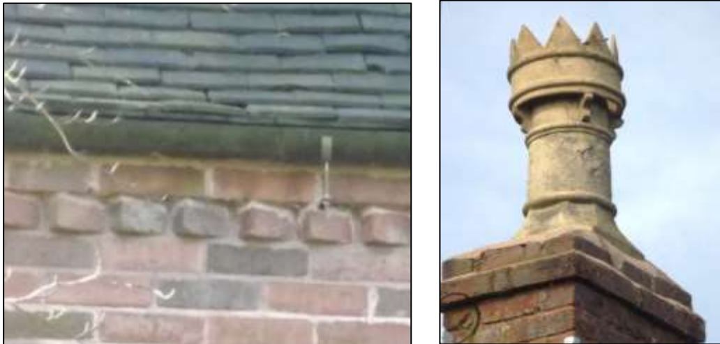
Figure 16: Dog-toothed eaves, castellated chimney pot and array of moulded brick chimneys at Hilderstone Hall
