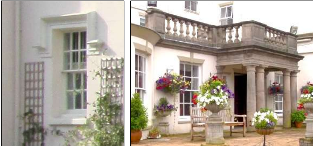
Figure 12: Hood mould over sash window within deep reveal at Hilderstone House, and elaborate portico with balustrade over door to Hilderstone Hall
