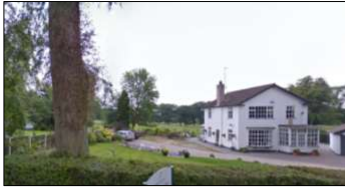
Figure 77: The character of historic buildings can also be harmed by simple alterations such as widening historic window openings
