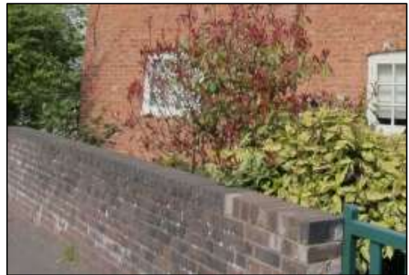
Figure 17: Variety of brick boundary walls with a variety of brick or stone copings
