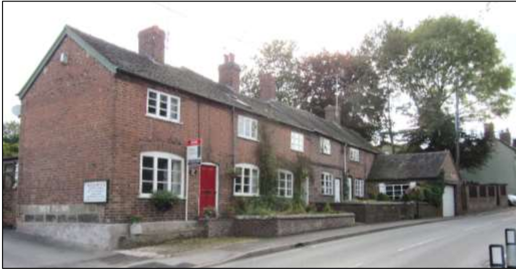
Figure 32: Hall Farm Cottages
