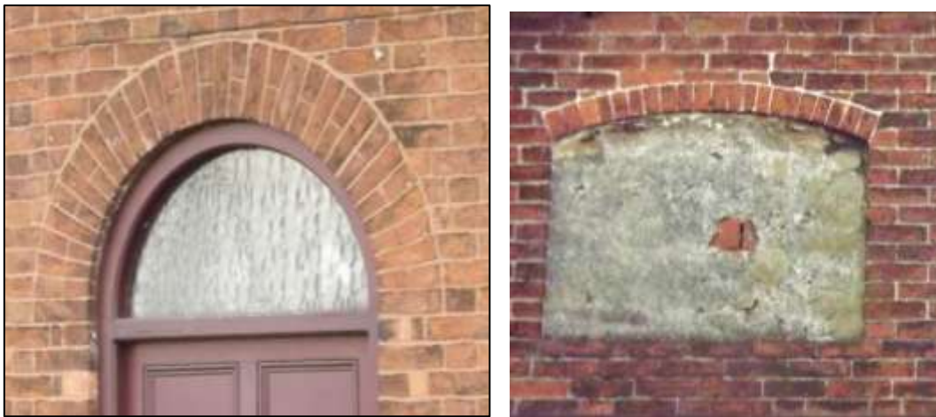
Figure 11: semi-circular brick arch over fanlight at Lower Farm house, and variations of the segmental arched window head.
