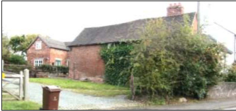
Figure 36: Plain functional elevation to side of Mill Cottages indicating former agricultural use, and further outbuildings to rear
